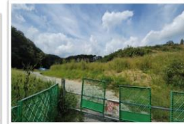
← Site of Otawara Solar Power Plant
